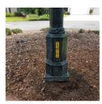
These numbers found on the light posts in Island West identify the location of the unit. If a bulb is burnt out or should the pole get damaged write this number down or take a picture like this one and Email or call IMC to report it. The electric company will then know where it is.....although a physical location is smart to add to your alert...such as 'across from 123 Yonges Is. Dr.'
